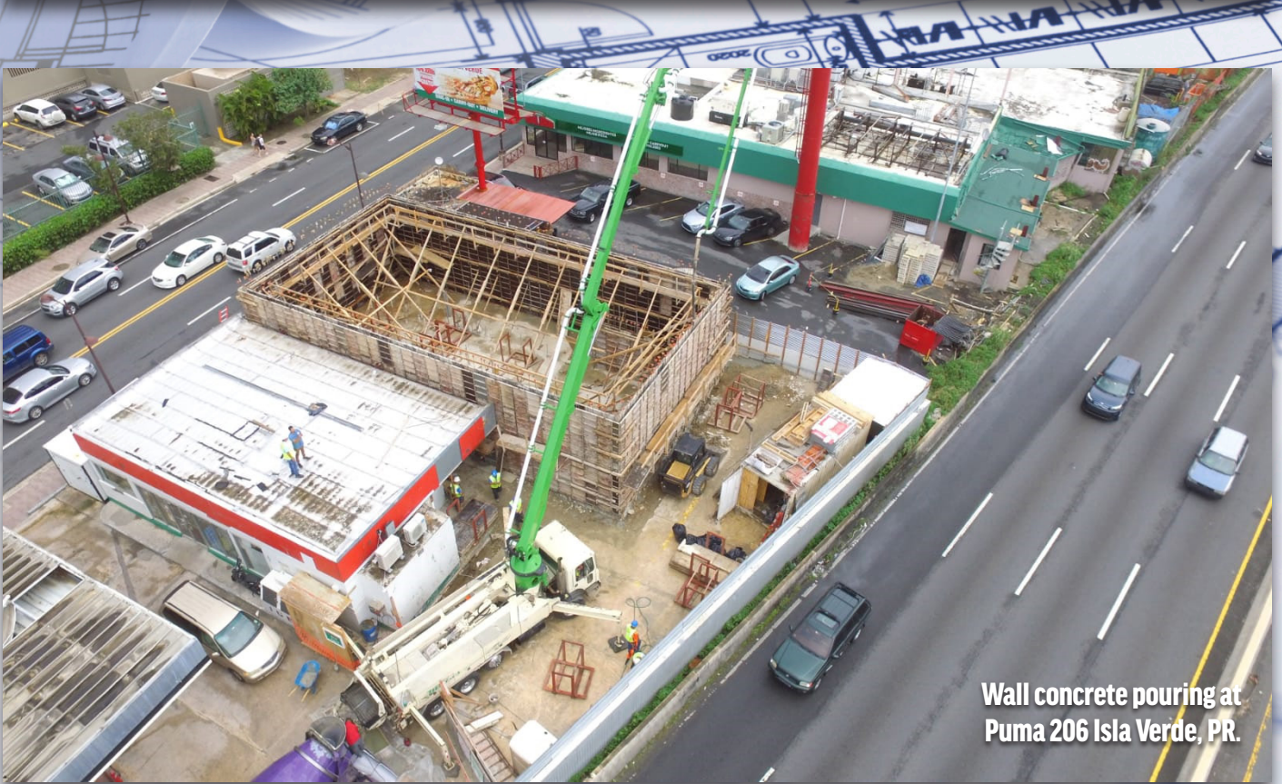
Construction of new Lares Coop branch location on PR 129.
